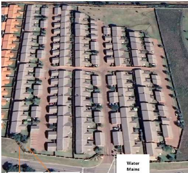
Borehole Bladder and Mains
